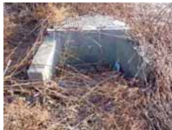
Outlet to Gravelly Run (buried)
